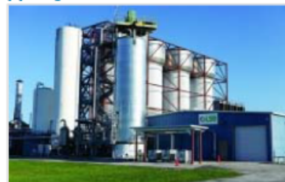
LS9 makes fatty alcohols at this plant in Florida.
